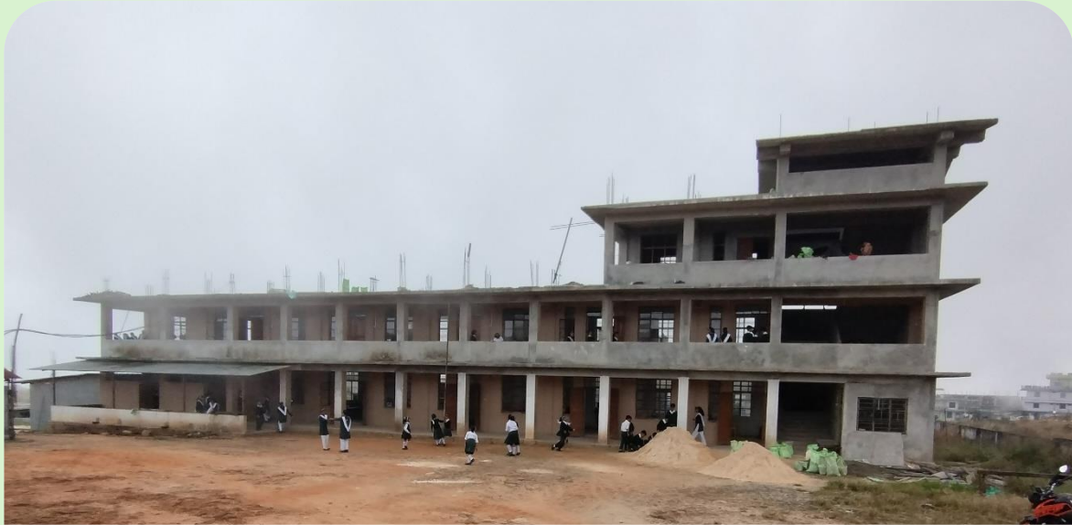
Mawsmai School under Construction
