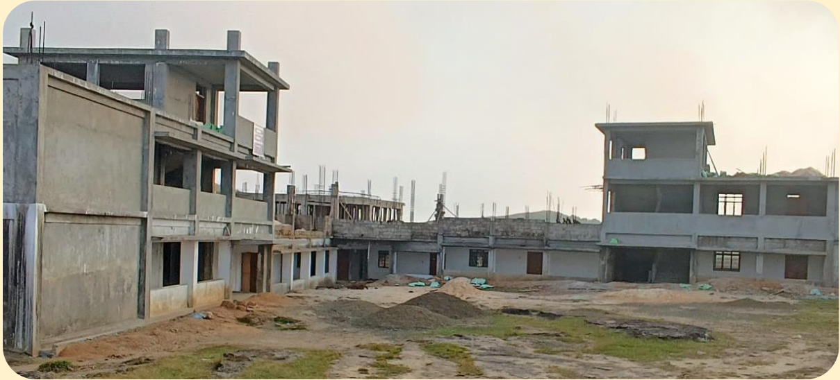
Lummaushken School under Construction
